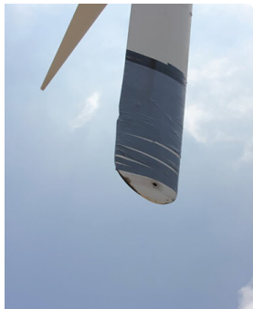
DAMAGE TREATED WITH ADHESIVE TAPE
